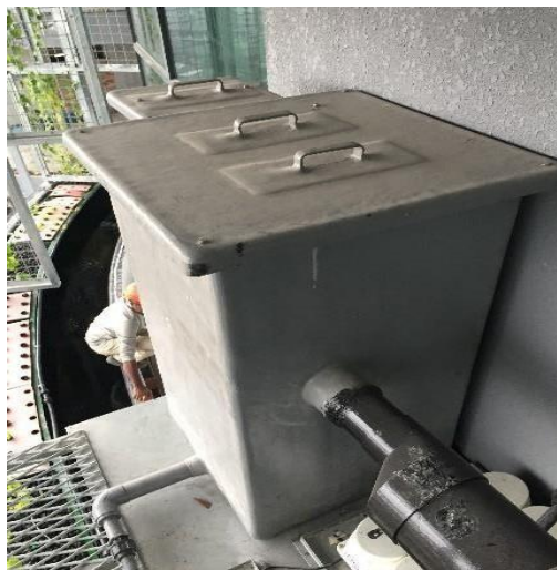
Figure 6 : Lamella Clarifier
