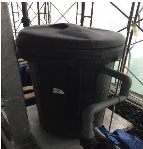
Figure 7 : Denitrification unit
