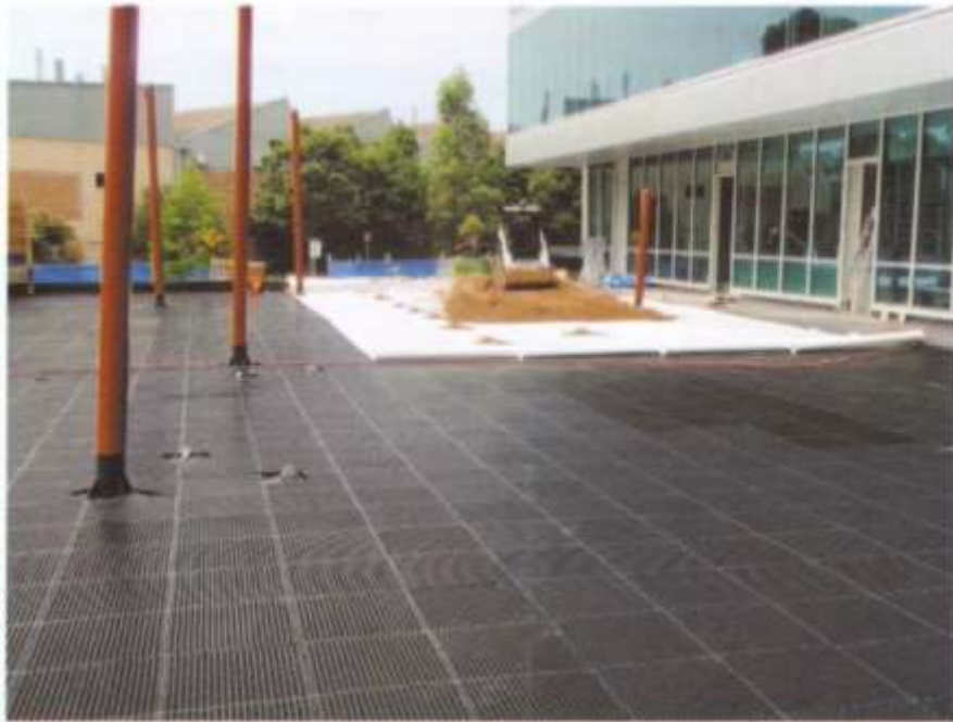
Drainage cell installation in progress.
