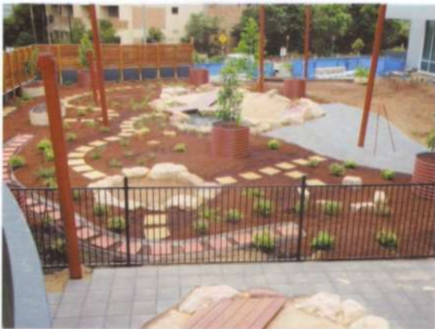
Construction of roof garden upon completion of drainage cell installation.
