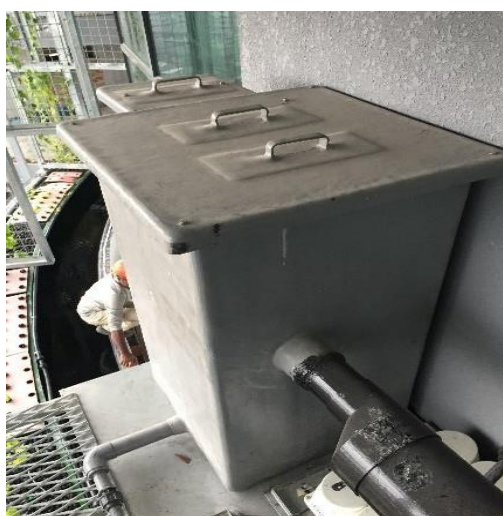
Figure 6 : Lamella Clarifier
