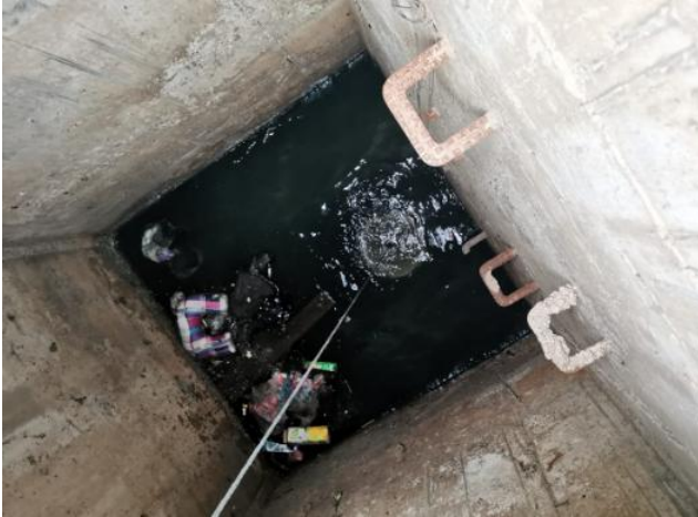
Blackish and smelly water at inlet sump
